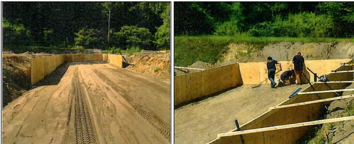
**Figure 4-4. Installing 45 mil pond liner inside the woodchip containment area; rolls 60 ft long by 10 ft wide**
