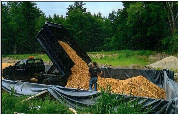
**Figure 4-7. More filling with woodchips and grading the interior**
