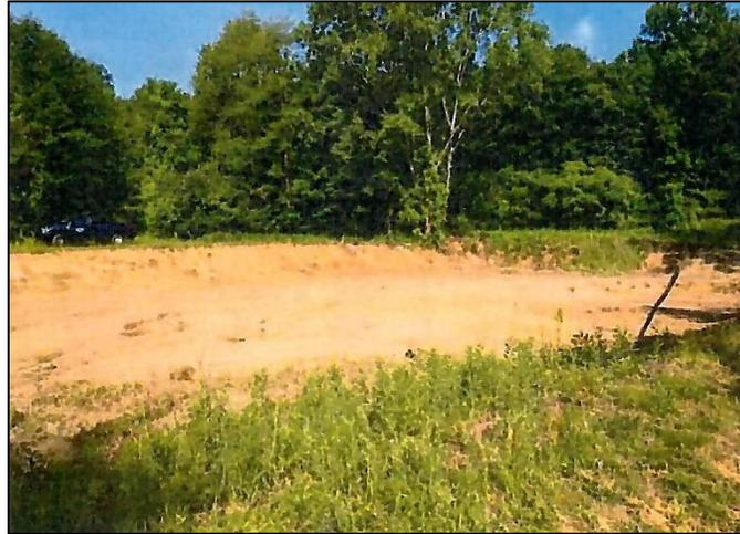
**Figure 4-2. Grading of the base of the woodchip bioreactor during installation**
