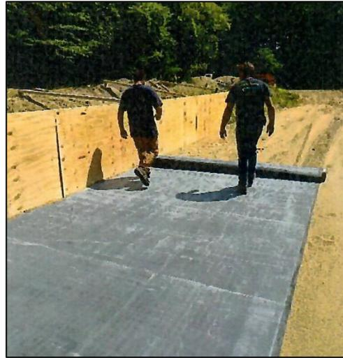
**Figure 4-5. Pond liner installed**
