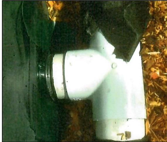
Figure 4-10. Filter fabric covers woodchips to protect from soil
