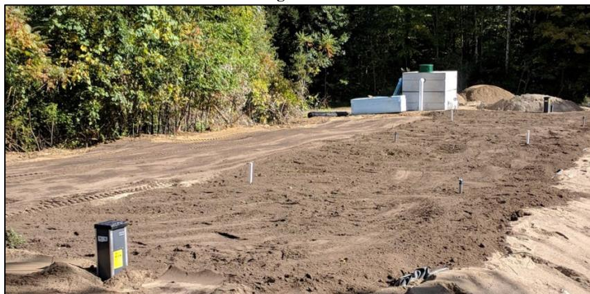
The *effluent* control structure is in the foreground of the photograph, with the *influent* control structure at the opposite end. The six (6) PVC *bioreactor monitoring wells* are shown installed at the 25-, 50- and 75-
